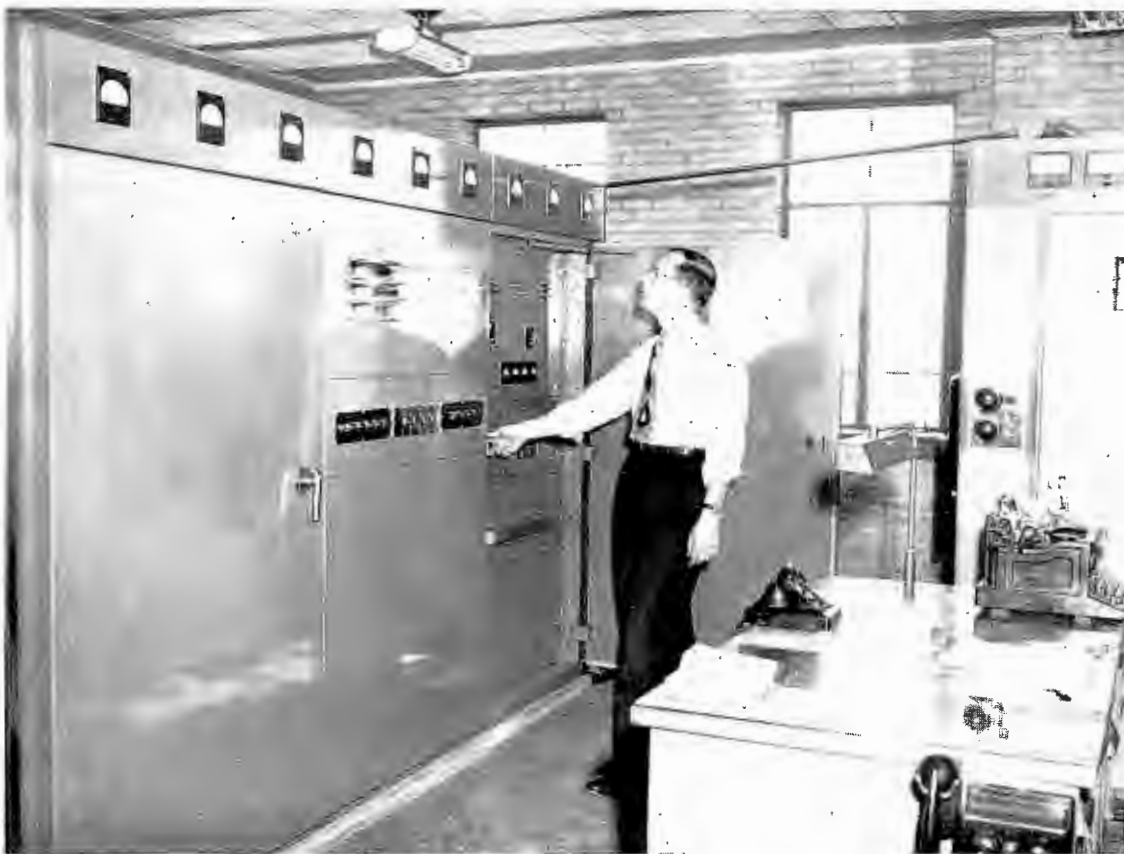
Above—BC-5B 5000 watt Gates broadcast transmitter installed at Radio Station WTAD, Quincy, Ill., CBS outlet and pioneer midwestern station.
